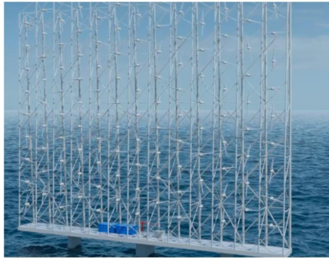
Figure 18-2 Wind Catching floating multi-turbine technology (30)
