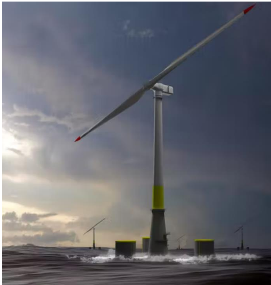
Figure 18-1 Seawind teetering hinge rotor design (29)
