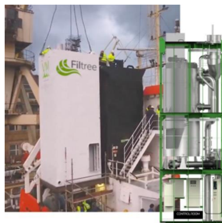
Figure 12-2 Filtree system being lifted in place
