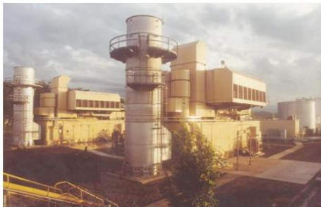
Chaco 90 MW OCGT BPs aeroderivative fleet for a gas field Bulu Bulu, Bolivia
