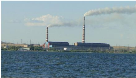
Karaganda GRES II 608 MW Coal Second largest coal fired plant in Kazakhstan
